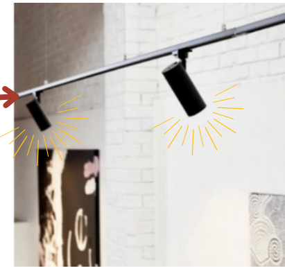
Suspended track with adjustable spotlights to illuminate artwork and corridor
